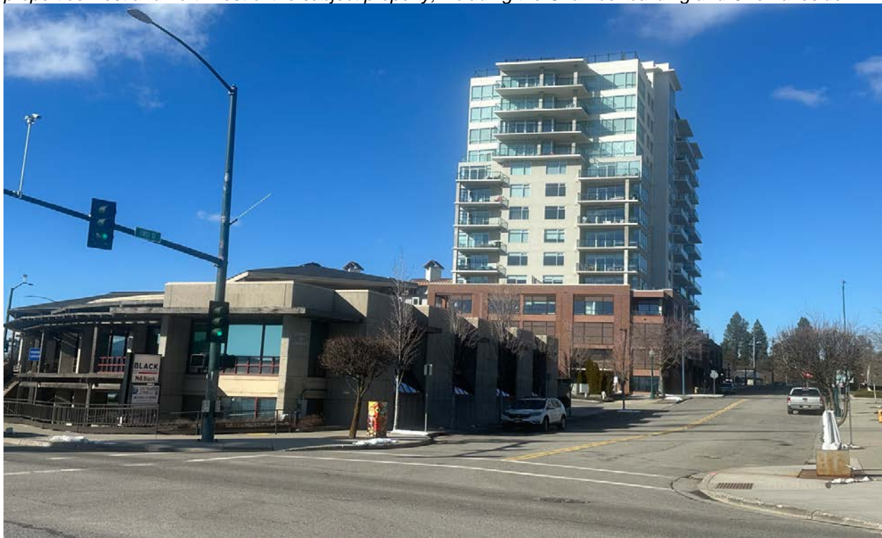
SITE PHOTO – 10: View looking north from the intersection of First Street and Sherman Avenue at the properties west and northwest of the subject property, including the Chamber building and One Lakeside.
