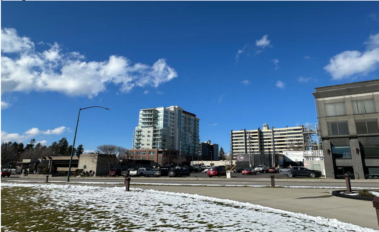
SITE PHOTO – 2: View from the grassy area in front of the Coeur d’ Alene Resort from the south side of Sherman Avenue looking northwest toward the project site which includes (right to left) the Johnson Building, parking lot, and the former MoMo’s restaurant.
