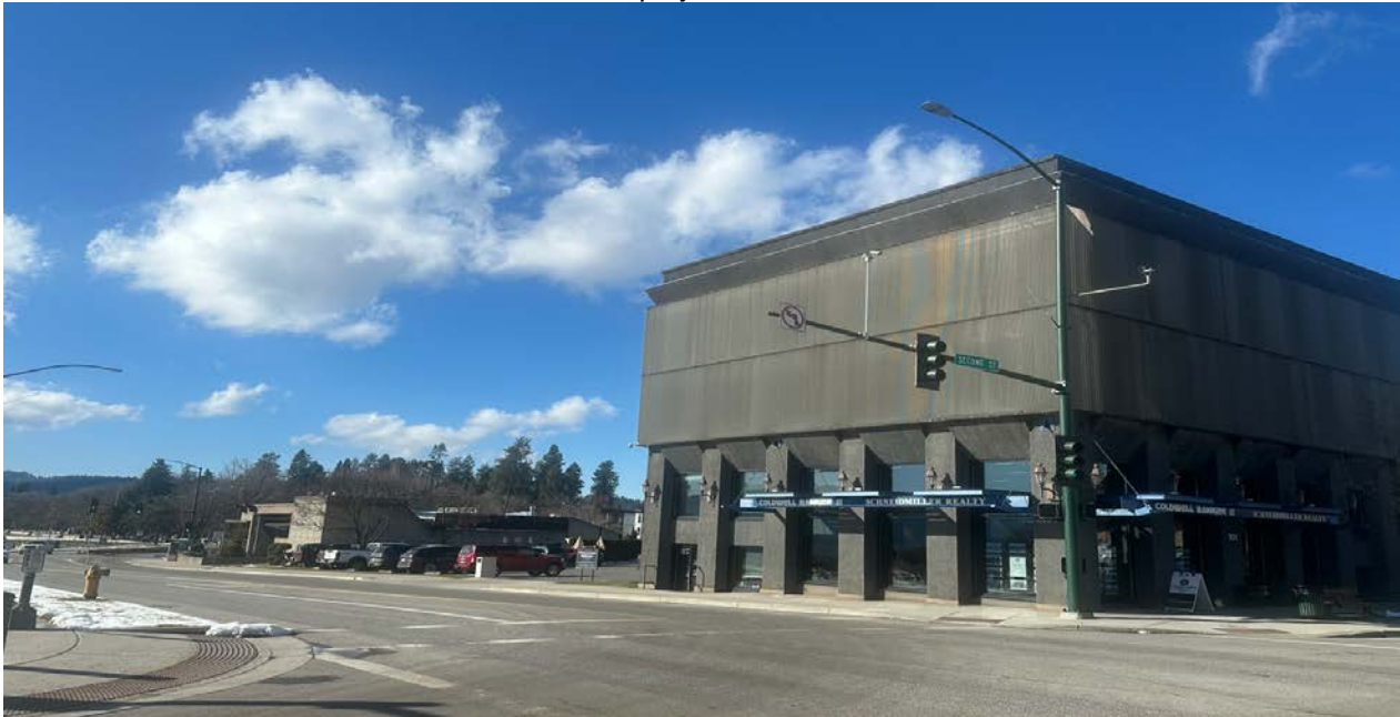
SITE PHOTO – 1: View from the intersection of 2 nd Street and Sherman Avenue looking northwest at the proposed site. There are two (2) existing structures on the site that will be removed including the Johnson Building and a former Momo’s restaurant on the west side of the project site.
